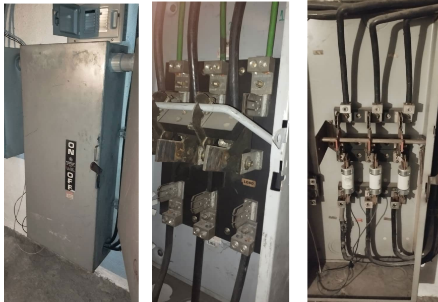
Figure 19 - Main Disconnect switch
