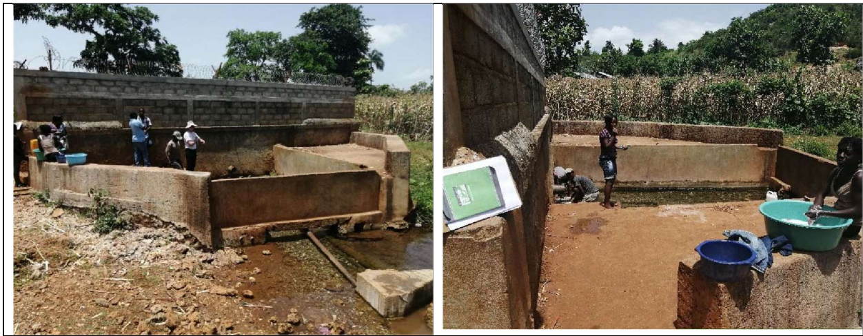
Figure 8. Discharge through orifice at base of cross wall (left) and entry to tailrace stairs (right)
