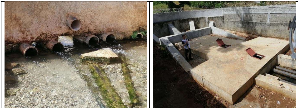
Figure 3. Overflow pipes at discharge on north side of enclosure (left); at exit of spring capture (right)
